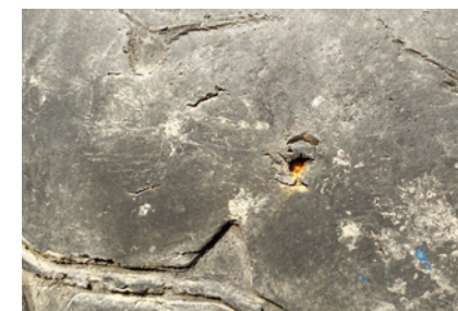
Inner tyre material is rusty
